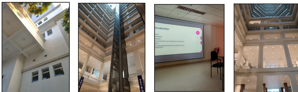
From left to right: Entrance to the new tower block of the faculty of medicine; View from the inner courtyard of the tower block; Excellent facilities inside the block; Inside view of the floors. Source: the author
